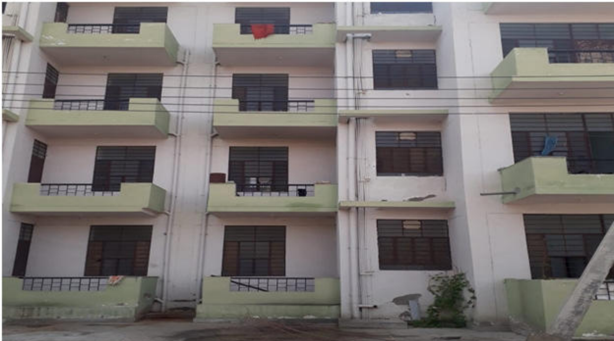
MIG-A (G+3) flats at Govind Nagar, Rajsamand
