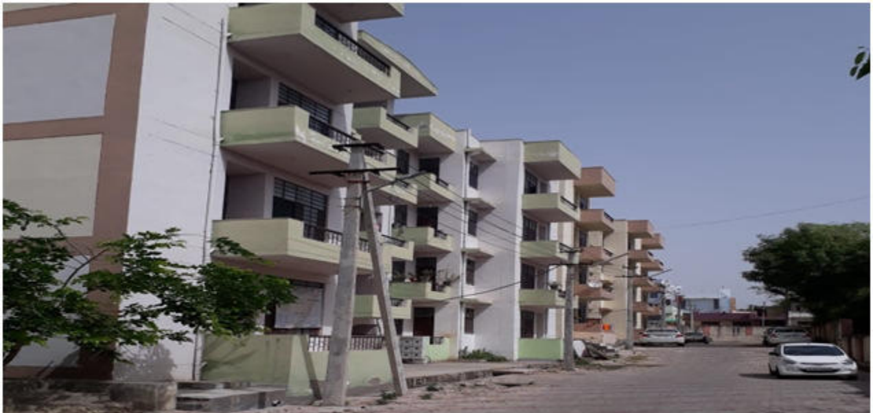
MIG-A (G+3) flats at Govind Nagar, Rajsamand
