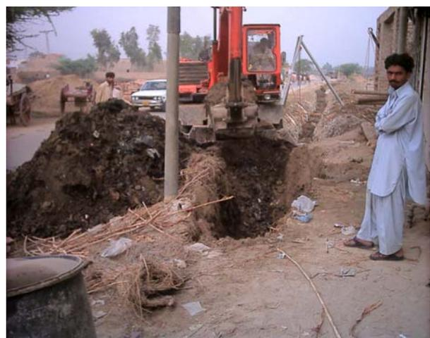
**Photo 18: Backhoe digger for trenching**
