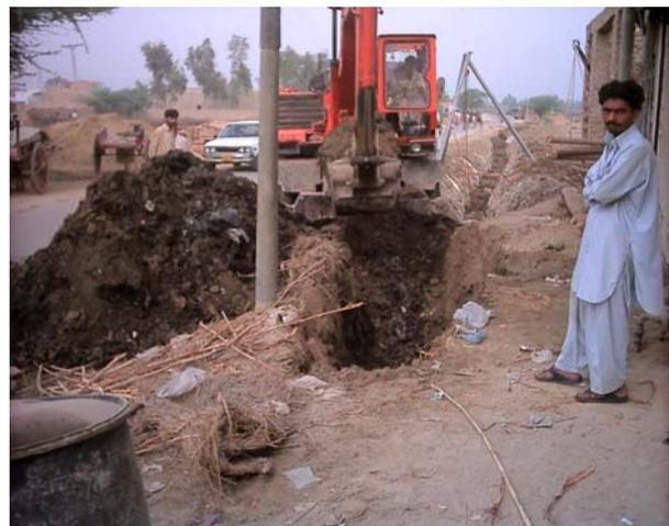
**Photo 18: Backhoe digger for trenching**
